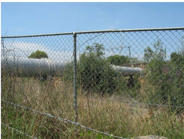
Photo 3.8: Upper Canal 'aqueduct' over the main southern railway. Photo taken from Mt Annan Botanic Gardens. February 2004
