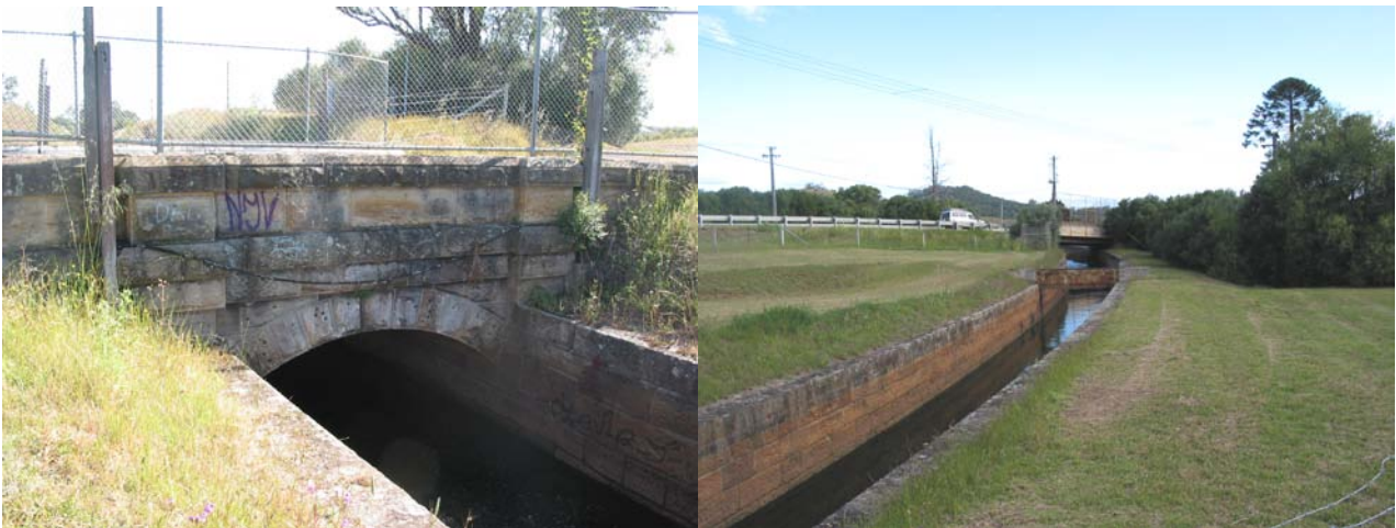
Photo 3.7: Glenlee Road crosses over the canal on this stone bridge (left). View to southeast looking to the Menangle Road bridge over the canal (right). November 2003
