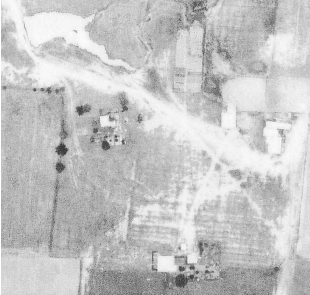
Figure 4.5: 1947 aerial showing two groups of building associated with this property. North is at the top. The northern group is visible on the 1888 plan. The southern group is in the same location as the stables on the 1888 plan (Fig. 4.6).
