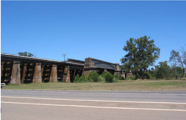
Photo 3.1: View to south east showing the Menangle rail viaduct and bridge. This items is on the State Heritage Register. November 2003
